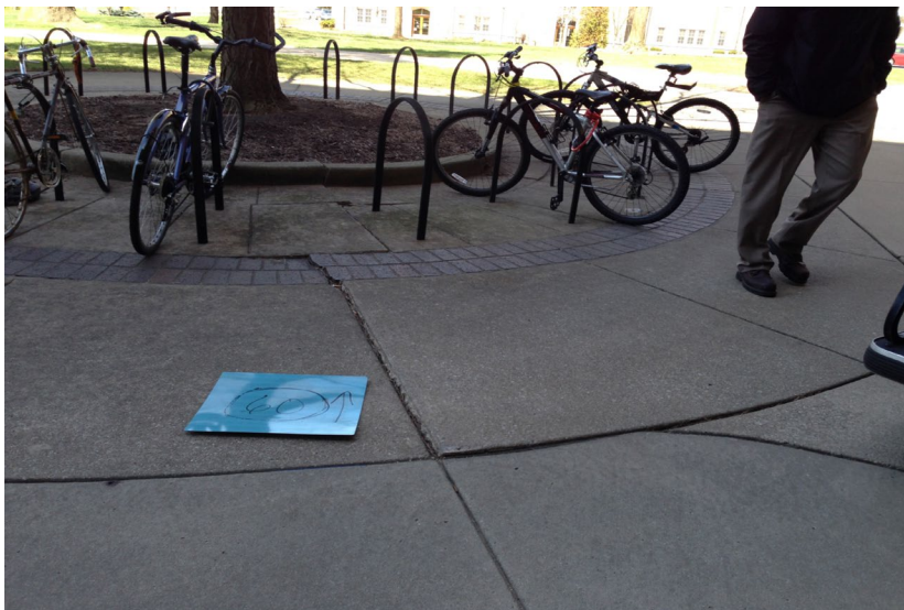
Picture 2: Level Changes at Sidewalk-to-Pavers
