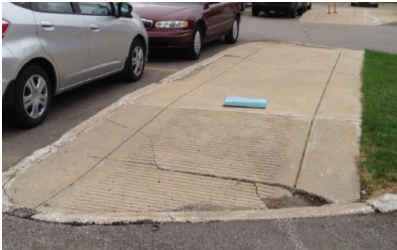
Picture 1: Curb Ramps
